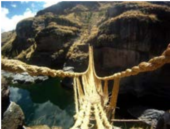
Inca suspension bridge. Made of grass.
