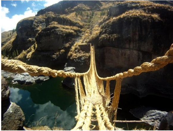
Inca suspension bridge. Made of grass.
